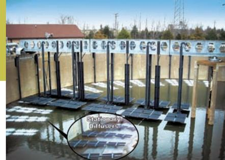
**There are 480 stationary diffusers mounted 8 in. above the floor on retrievable rack assemblies attached to the tank wall.**
