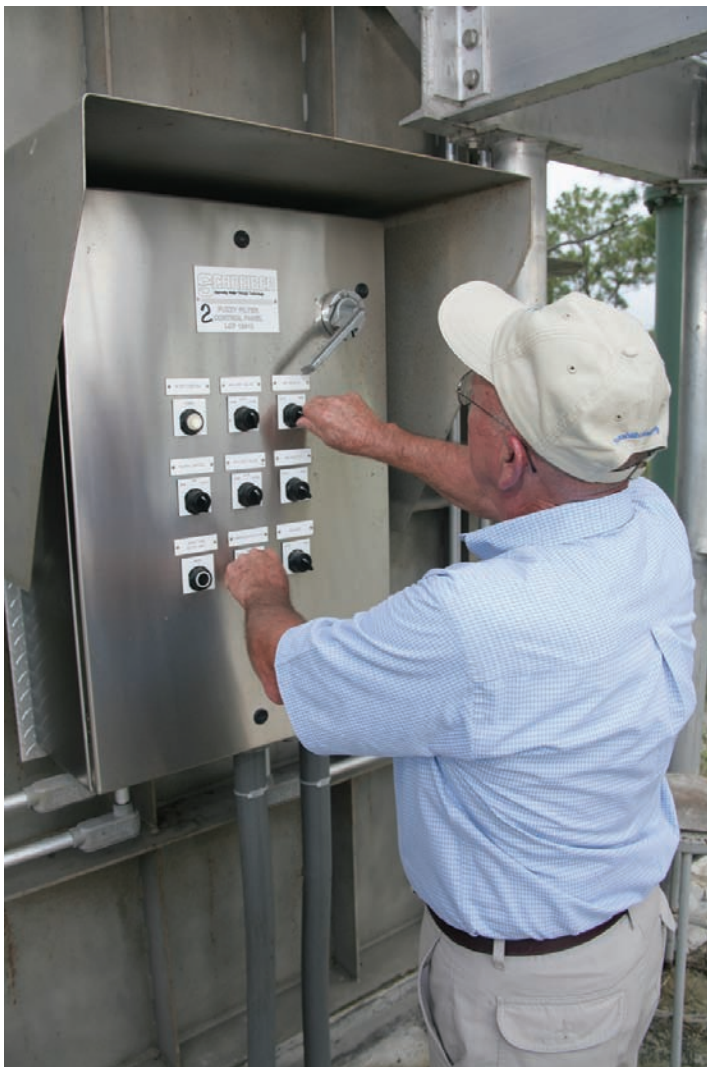
At the Schreiber control panel, Director of Operations Tom Vaughn can adjust the filter porosity or set the automatic washing.
