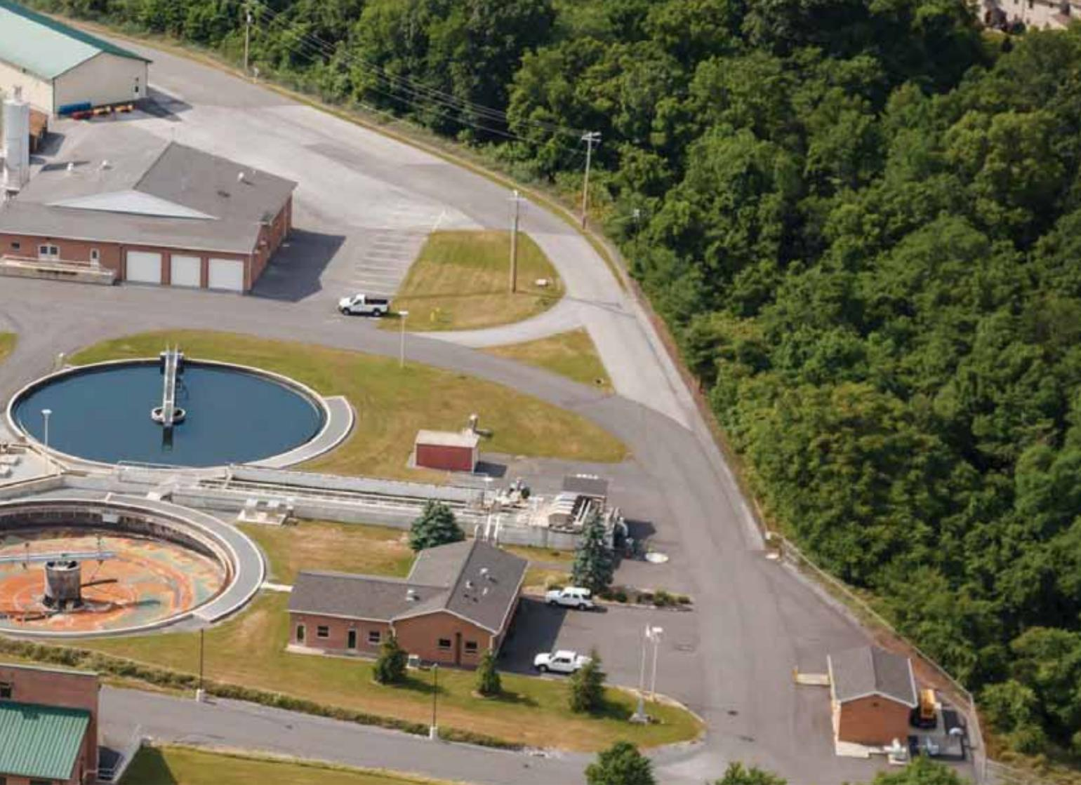
m<sup>3</sup>/d (6.78 mgd). The facility was constructed in 1982 and upgraded in 2010. It consists of five influent wastewater screens, a spiral-flow aerated grit and grease removal system, two CSR basins, three final clarifiers, and ultraviolet disinfection.
