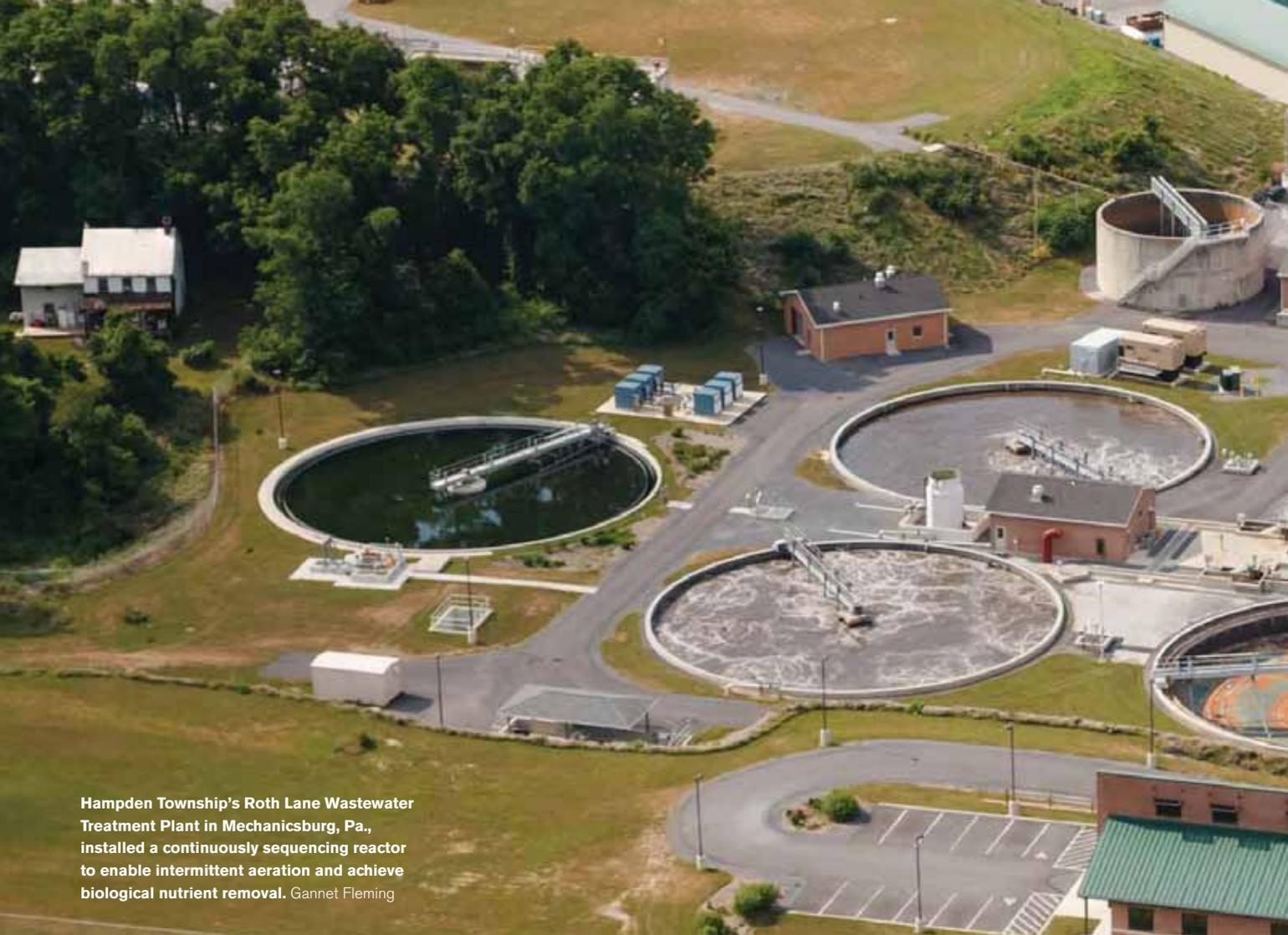
Hampden Township's Roth Lane Wastewater Treatment Plant in Mechanicsburg, Pa., installed a continuously sequencing reactor to enable intermittent aeration and achieve biological nutrient removal. Gannett Fleming
