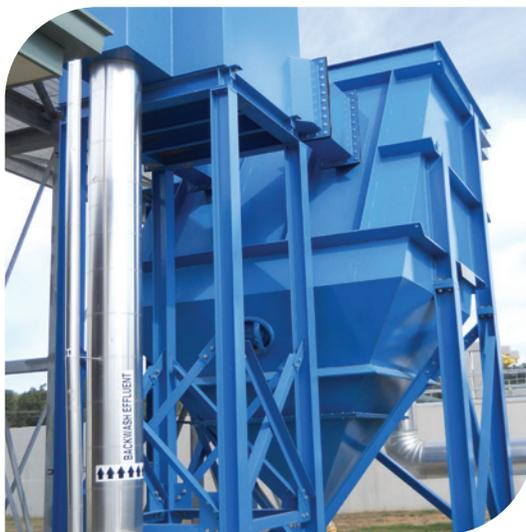
The clarified liquid leaves the plate assembly through orifices or weirs at the top and is distributed into collection channels leading to the clarified water outlet. This creates a pressure drop across the collection channels which ensures uniform flow distribution across the plates in order to utilize the full area for settling.
